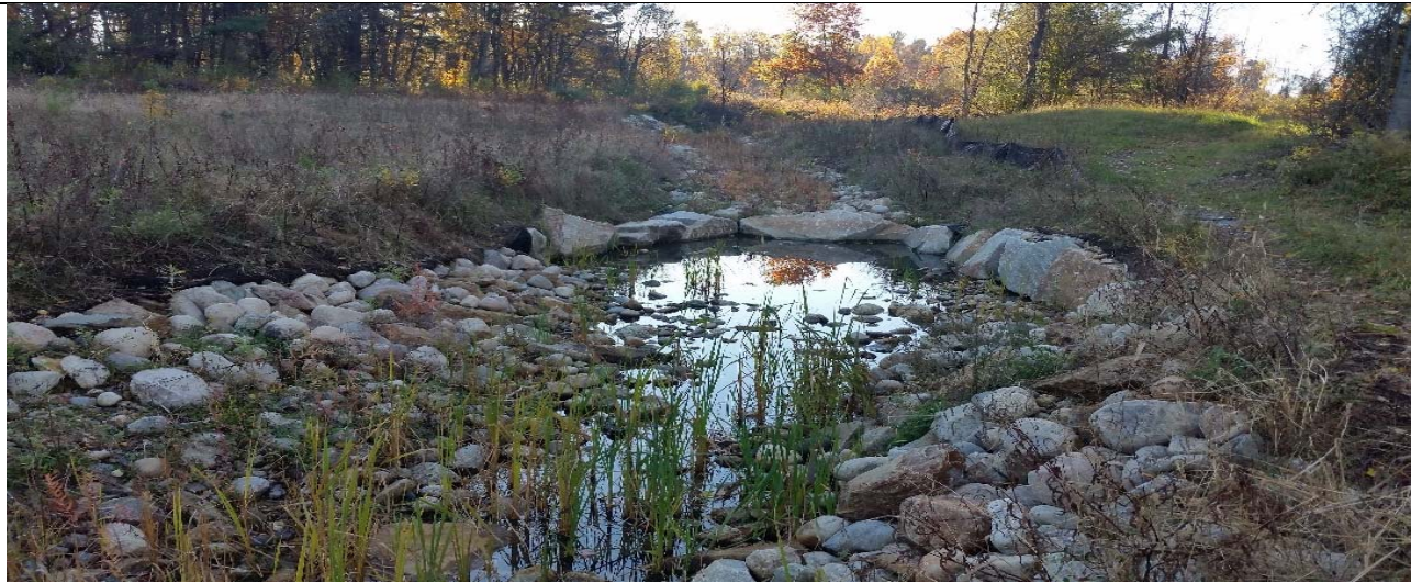
Photo #2: Sta. 7004+25 – Looking Upstream
