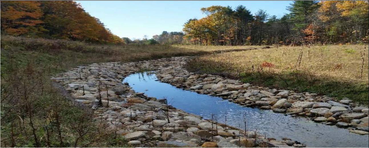
Photo #8: Sta. 7021+25 – Looking Upstream
