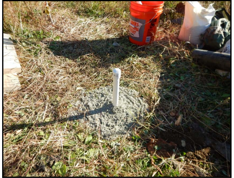
Shallow Groundwater Well #1 installed within Zone 2 along the eastern side of Railway Brook adjacent to Stations 7005-7006. Date: 10-23-2015.
